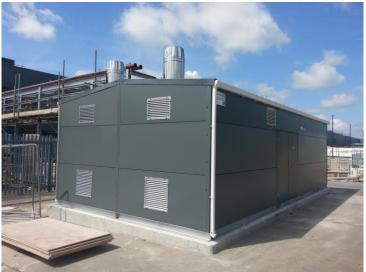
LPHW Plantroom with 2 no. 1500Kw Rendamax high efficiency boilers serving a Low Loss Header with 3 no. Heating circuits
